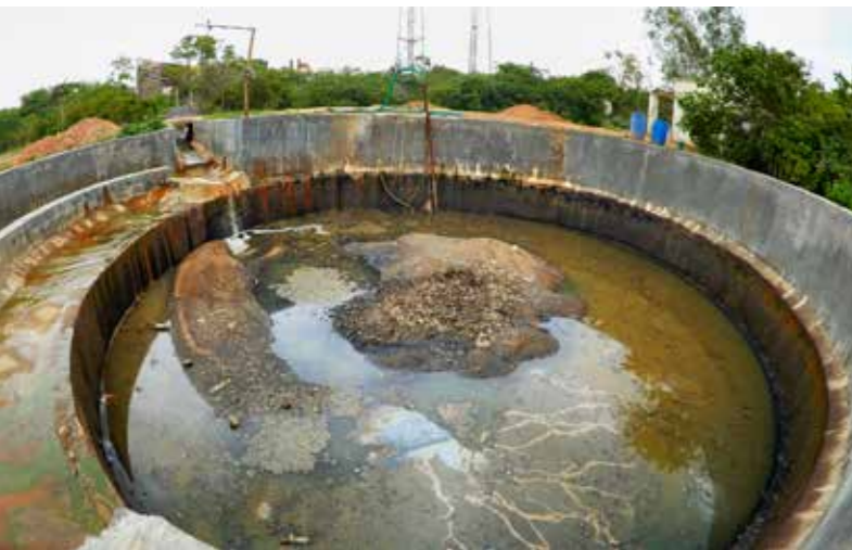
A circular effluent tank at Gadapotharam industrial estate, collecting effluents from nearby pharmaceutical factories. The tank is completely open and exposed.
